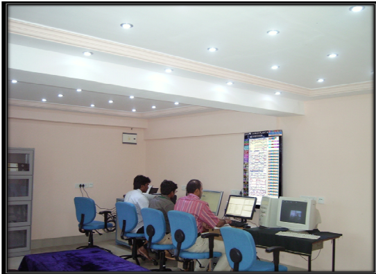
Fig. 1.8 Central Monitoring Unit
