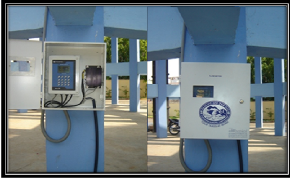
Fig 1.2 Installation of flow meter
