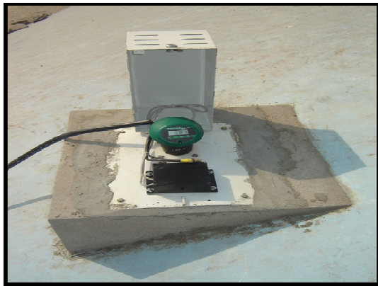
Fig. 1.3 Installation of digital level meter
